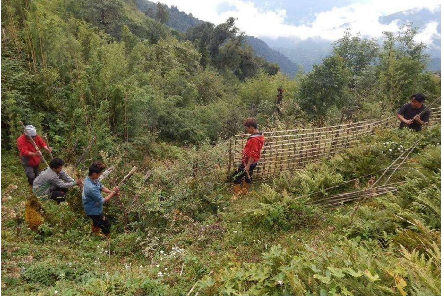
Bamboo mesh strip fence installation at restoration site in Jaubari, Ilam, eastern Nepal.
